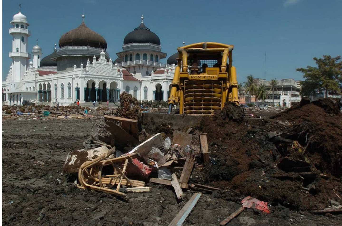
PHOTO BY HOTLI SIMANJUNTAK (ABOVE) PHOTO BY AGUS SUSANTO
